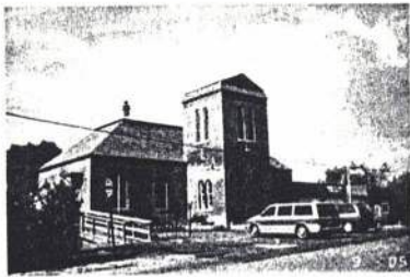
Village Hall –Pine Street
