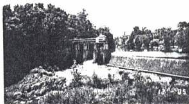
Fish Creek - On Bridge Street looking South
