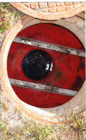
Fig 7 View over center shaft into sediment storage zone.
