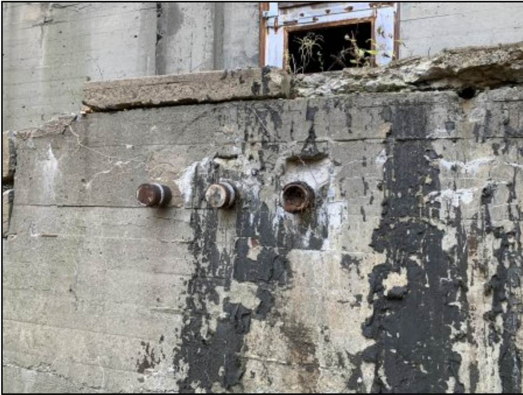
View of tar traveling down structure into deposit area.
