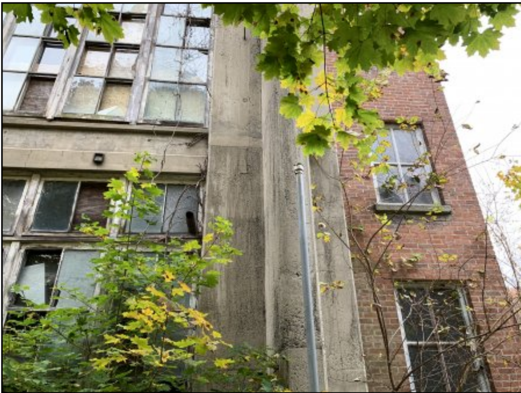
Vent line observed in northeastern corner of structure.
