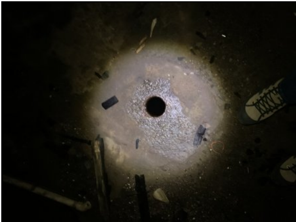
View of penetration in concrete slab of basement.
